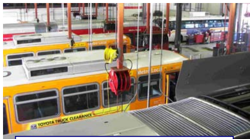
LA Metro Bus Maintenance Facility
