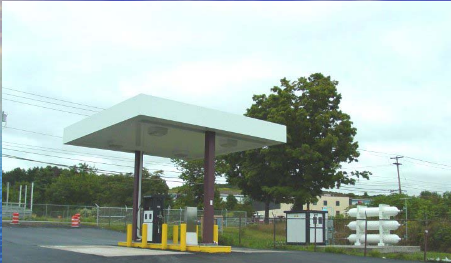
BARLOW ROAD, BINGHAMTON CNG SITE, REGION 9 - 3 SEPT 03
